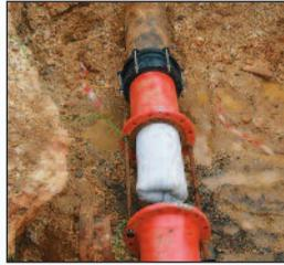
InsituMain® is installed inside the existing host pipe, eliminating the risk of disrupting or damaging any nearby utilities or underground services. The trenchless installation method reduces the social and environmental costs of pipeline renewal projects by minimising the carbon footprint, site noise, traffic diversions and safety concerns that are present with traditional dig and replace methods.
